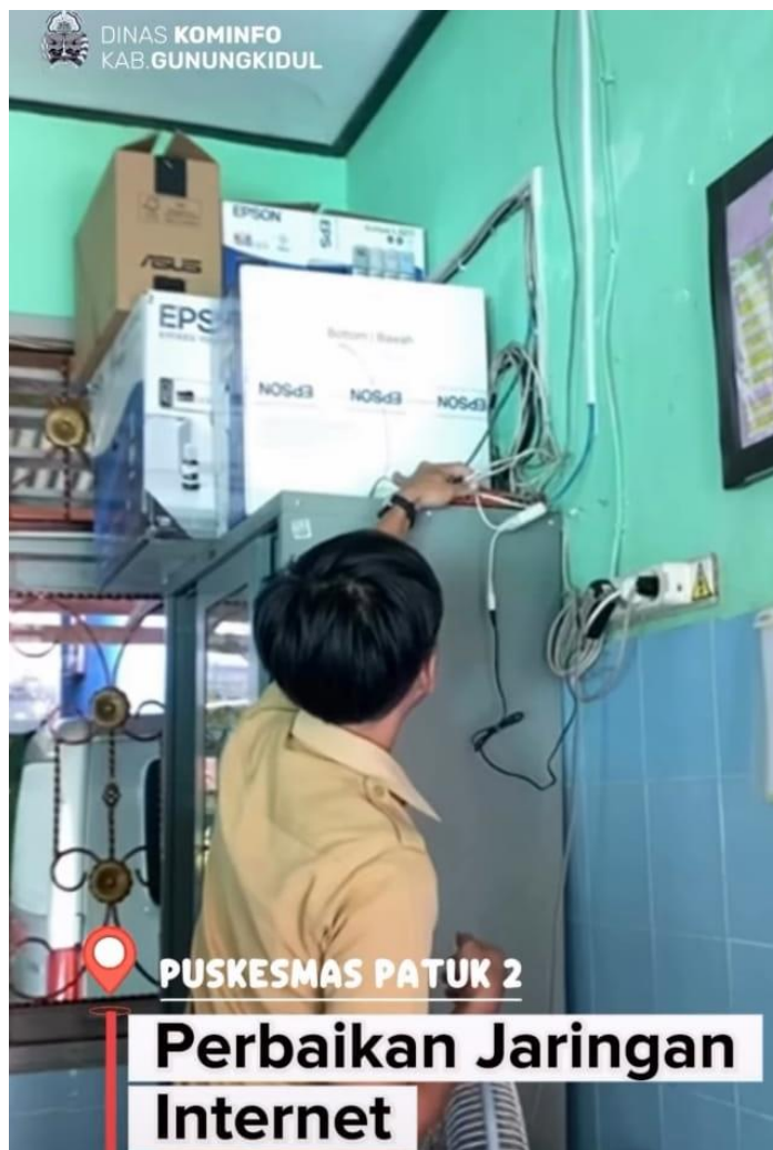
Gambar III.8 Perawatan dan Pengecekan Fungsi Peralatan
